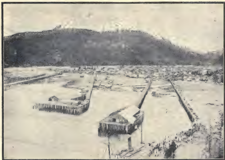
FIG. 166—The Docks at Skagway
